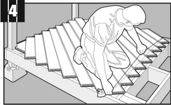
4 Snap a chalk line on all edges to indicate final cut length.
